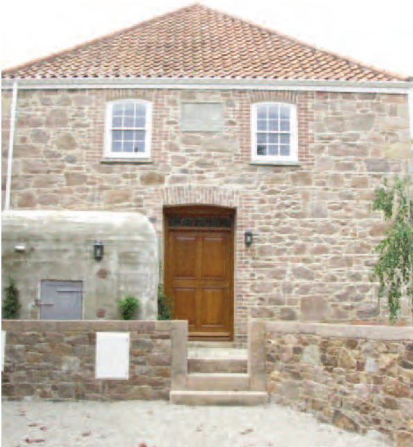
Front of chapel showing German telephone exchange to left
