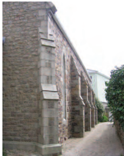
Side elevation showing buttresses framing lancet windows.
