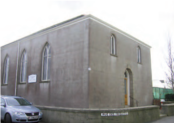
Eden Chapel from north west. Note the later nineteenth century cement-based render, and the 2-light Y-tracery windows which date from the late nineteenth century or possibly later.
