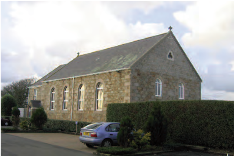
Bethlehem from south east, showing the structural break along the east entrance gable which indicates the conversion of the original hipped end into a gable.
